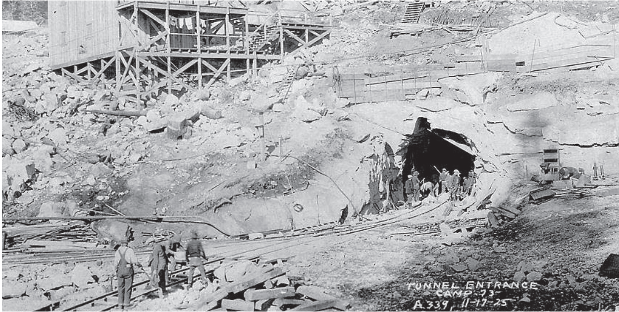
Camp 73 Tunnel at Big Creek, Nov. 17, 1925.
